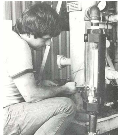
Jay Morris checks a pipe fitting on a sour gas plant being donated to the University of Oklahoma by Perry Gas Processors Inc. Morris rebuilt the plant to fulfill master's thesis requirements, and his efforts will enable OU students and researchers to search for effective methods of purifying natural gas.
