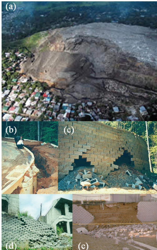
Figure 2. Example failures of geosynthetic structures: (a) A landfill failure in the Philippines resulting in 30,000 m 2 of debris, 200 deaths and hundreds more missing people 4 , (b-e) Failed MSE structures (Photos courtesy of R.M. Koerner and R.J. Bathurst). Development and installation of health monitoring systems in such structures could help prevent future failures and disasters.
