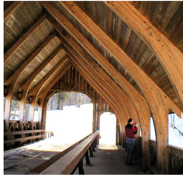
Inverset™ bridge with laminated timber beams
