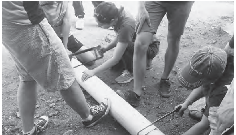
Melody Metivier Jones cuts slots in the casing pipe to be used in the new water well.
