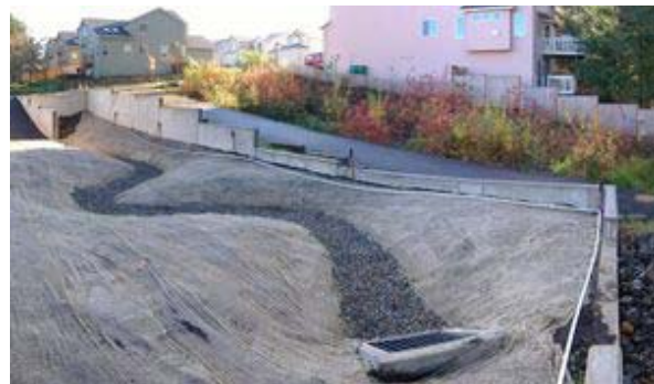
Bioswale being constructed in the foreground. Completed bioswale in the background.
