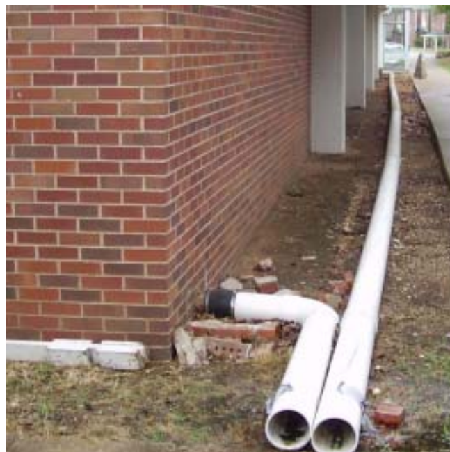
Pipe to move water away from the foundation of the library.
