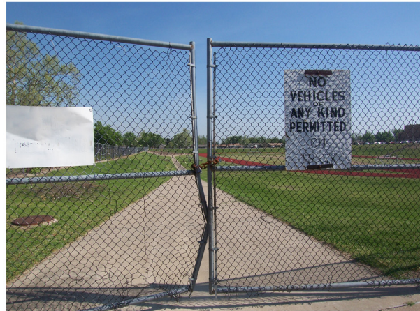
Vehicular Gate in Disrepair
