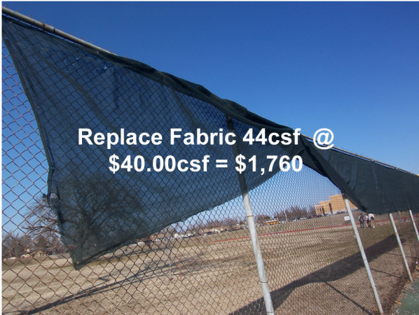
Turner Park Tennis Wind Mesh Repair Area
