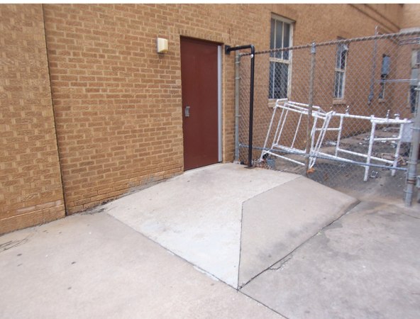
ADA Ramp is Non Compliant at Entrance
