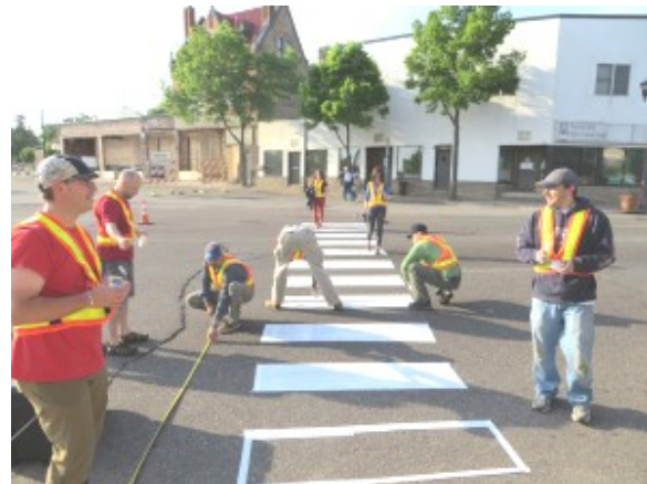
Volunteers installed a crosswalk and narrowed the crossing with bulbouts to improve safety at a midblock crosswalk.
