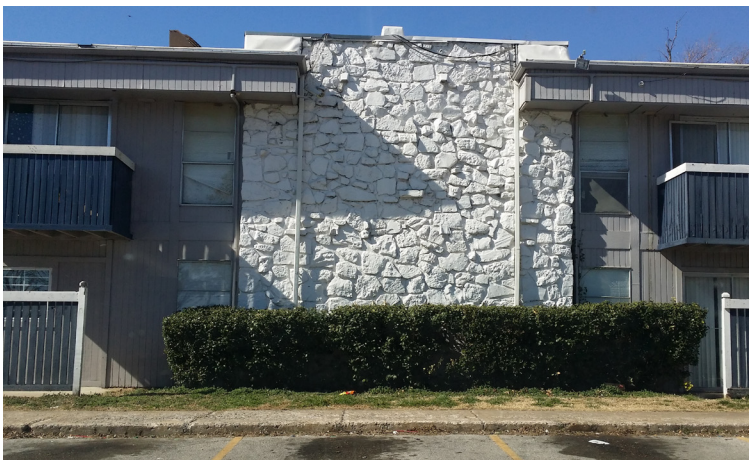
ABOVE: PALAZZO PARK. OVERGROWN HEDGES, ALTHOUGH NEATLY TRIMMED, ARE COVERING ANY CHANCE OF AN OCCUPANT ESCAPING THROUGH THE WINDOWS IN CASE OF A FIRE.
