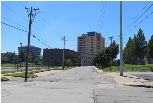
Paving and curbs are in poor condition and sidewalks are discontinuous and inaccessible
