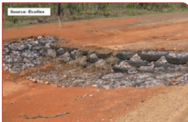
Figure 13.25: Weir made of rock-filled old truck tyres (source: Ecoflex)
