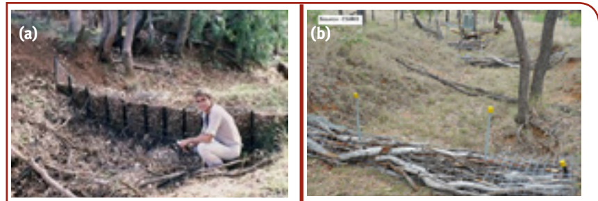
Figure 13.23: Field examples of wire netting weirs: (a) sediment trap used to encourage vegetation in the gully floor; (b) a variation—sticks and small branches or rocks, wrapped in wire netting, secured to the gully floor with stakes (Source: Wilkinson et al. 2013)
