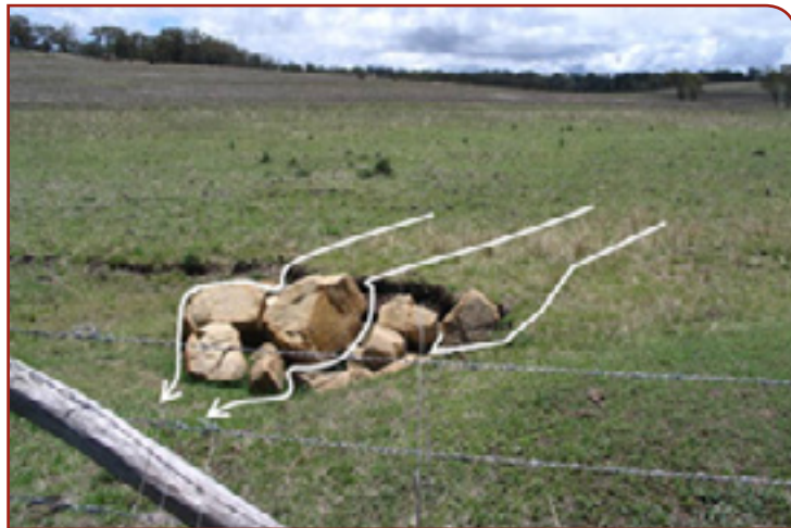
Figure 13.47: Haphazardly placed rocks fail to control erosion
