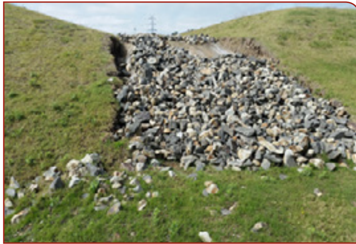
Figure 13.48: Field example of a failed rock chute; sidewalls not stabilised; geofabric used, but no wire netting to hold the rocks in place
